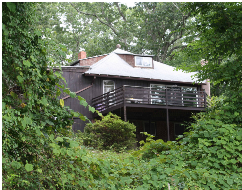
376 Kitemaug Road, Uncasville (Montville)
