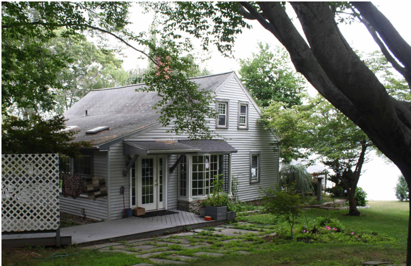
351 Kitemaug Road, Uncasville southwest view toward Thames River view
