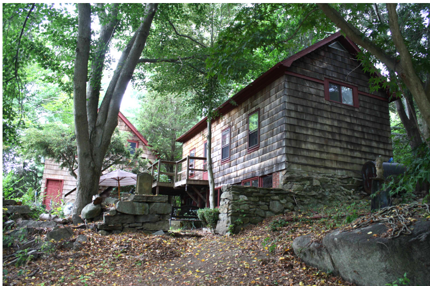
337 Kitemaug Road, Uncasville. Southwest view of Building I
