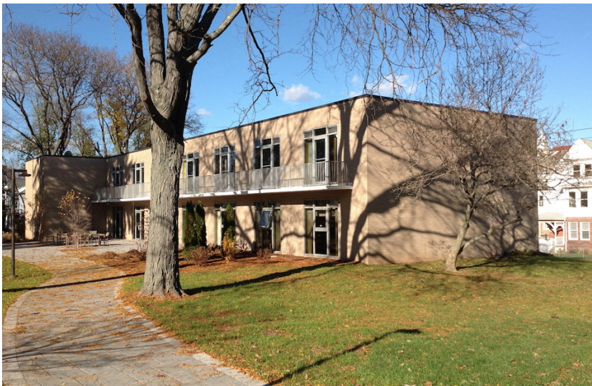
Center for Advanced Studies, 95 Pearl Street - southwest view
