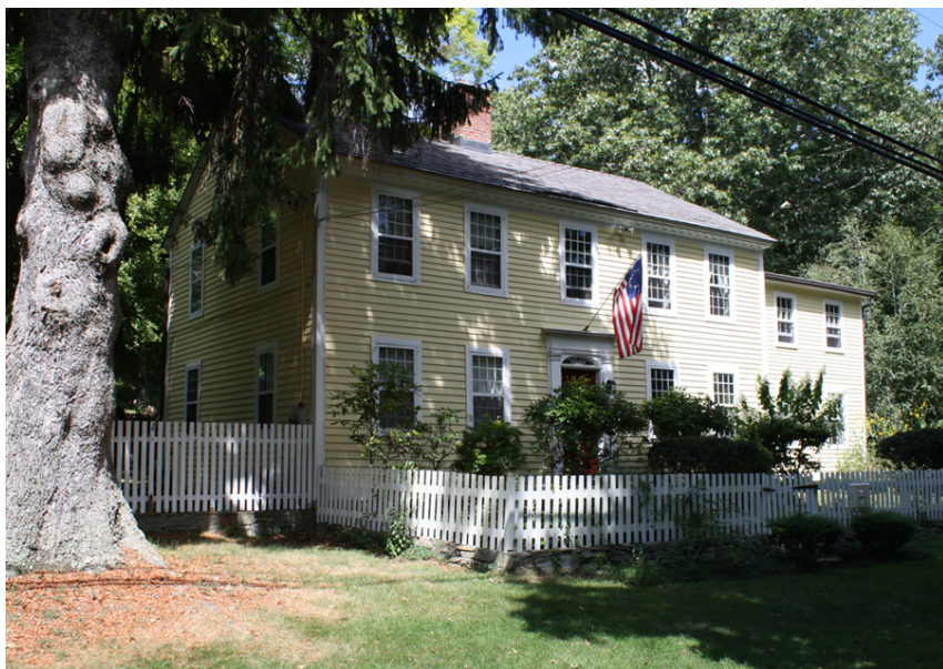
SW view of 76 River Road, Killingworth
