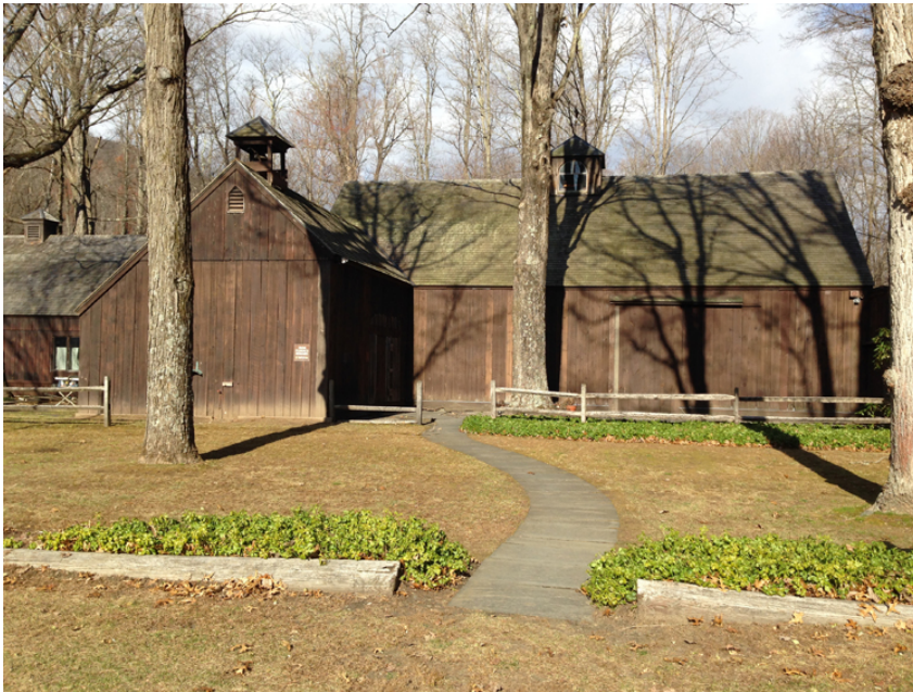
South side (facade) of the barn, camera facing north.
