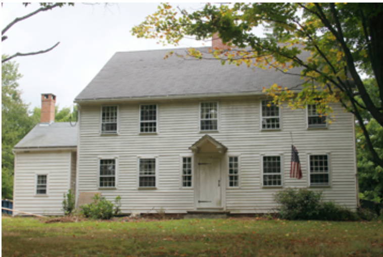
West view, camera facing east
