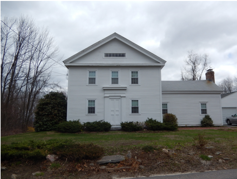
136 E. West Hill Road, Barkhamsted - West view
