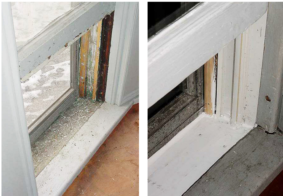
FIGURE 11.3 Window before and after friction treatment.
