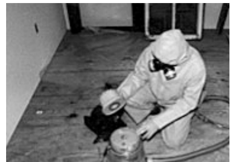
f) Remove & Replace HEPA Filter Assembly.
