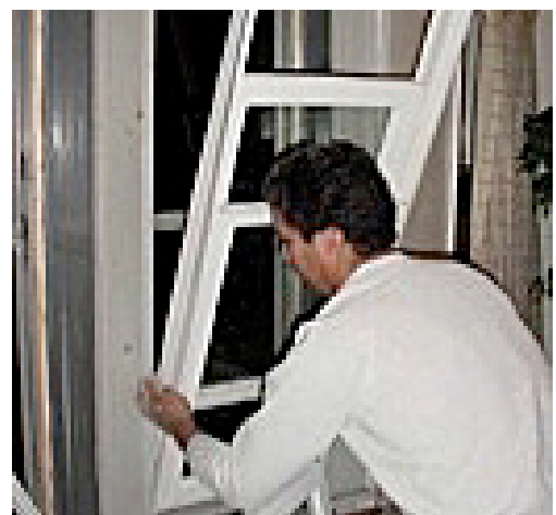
Figure 11.14 Reinstall sash into jamb.
