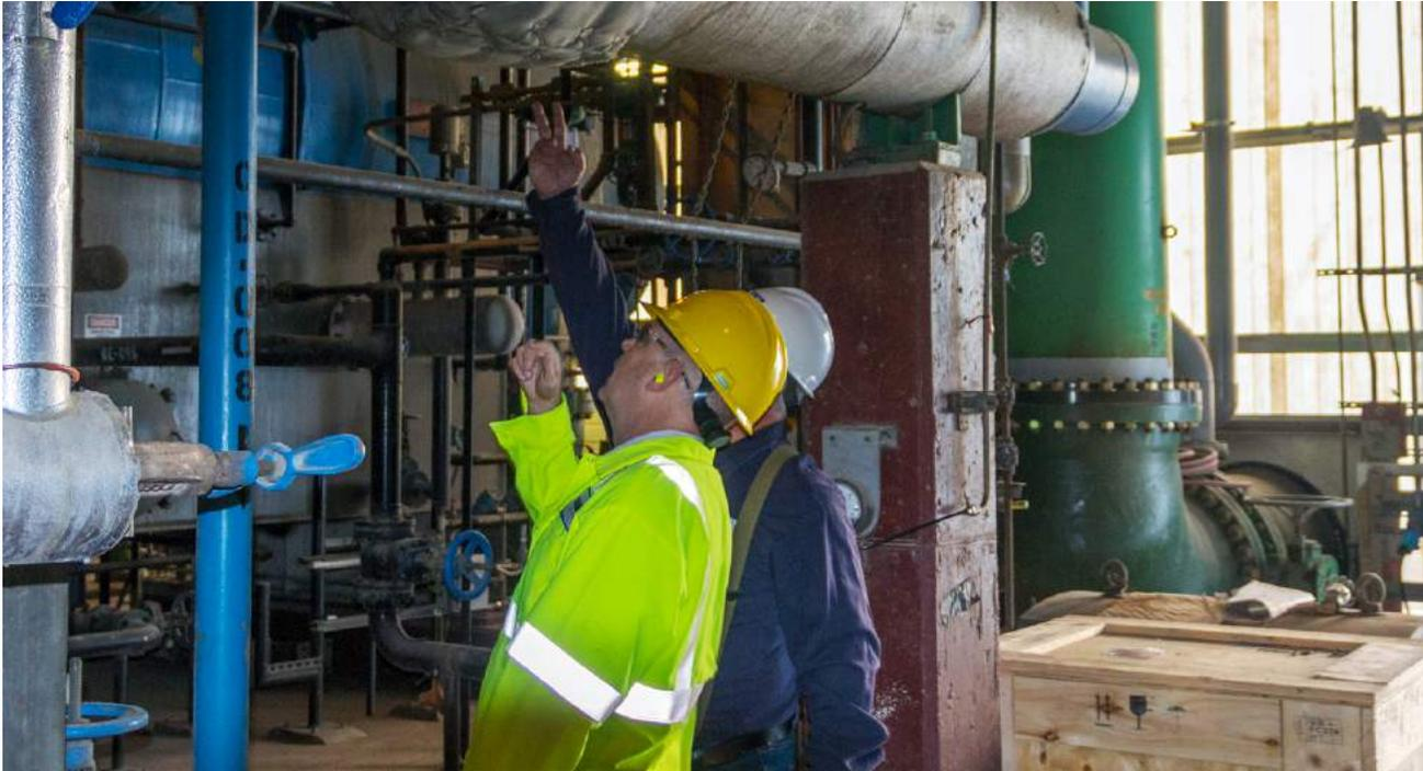
Covanta engineers at our Lancaster facility noticed that manually controlled water drain valves were being left on longer than necessary during plant start-ups, as operators tended to other tasks. Installing new automatic shut-off valves reduced the amount of water that drains to the sewer during start-up by 90 percent. Since the initial installation in 2015, this technology has now been installed at roughly three-quarters of our facilities.
