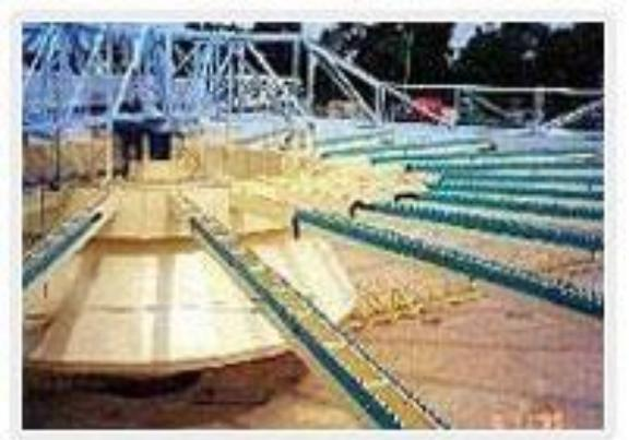
***View of the previous basin shown when empty to illustrate solids contact structure and bottom solids collector arms.***
