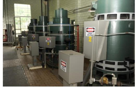
***Large pumps are used to transfer water from underground reservoirs and into four arterial mains that are 2-4 feet in diameter.***
