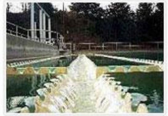
***The collection of water in weirs in the clarification basin after additional detention time has allowed more suspended particles to settle.***
