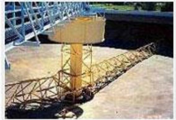
***An empty East Plant sedimentation basin shows large sweeps and blow-down structures used to collect and dispel settled solids.***
