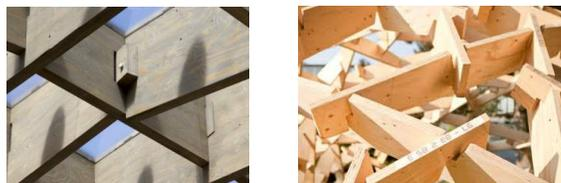
Figure 4: Mortise and tenon of the Serpentine Gallery Pavilion (Balmond [1]) and notching system designed by Thönissen [12]
