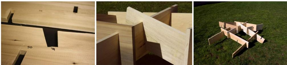
Figure 19. Framework built with rectangular boards
