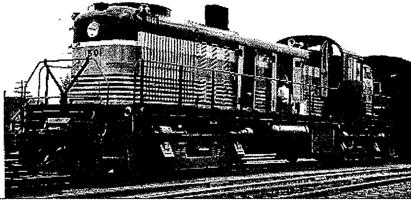
Montreal Loco Works 1501 RS2 demonstrator testing with CP dynamometer car on ONR 1949
