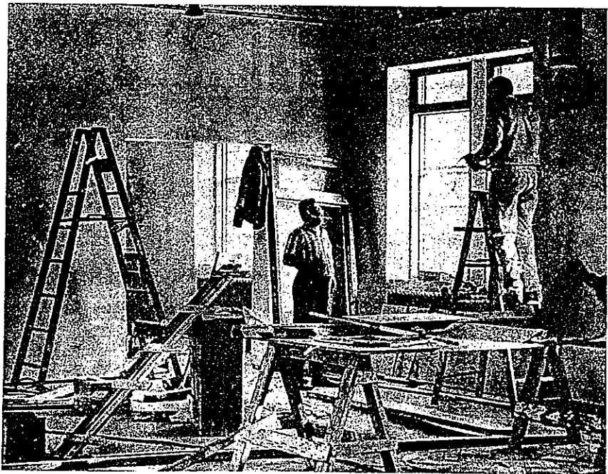
Timmins will boast one of the most modern stations in Ontario when work has been completed on a new waiting room, washrooms and office. Above photo shows carpenters on the job early in November.
