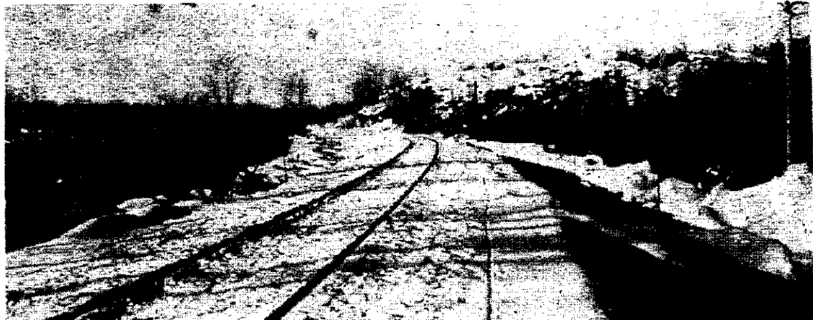
A Section of Track on the C.P.R. New Branch Line Between Havelock and Nephton, Ont.
