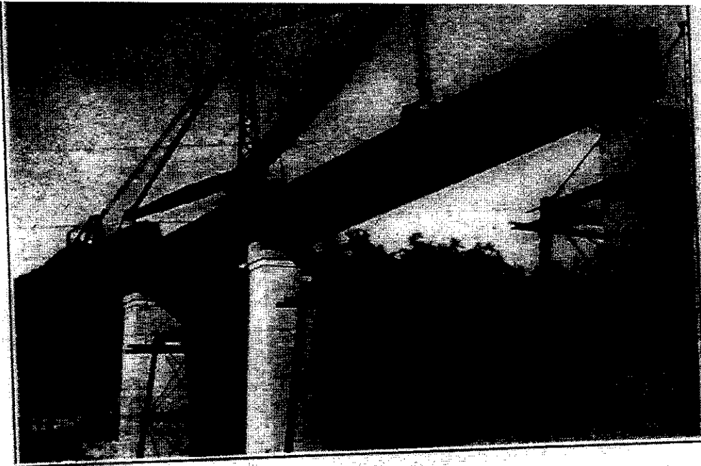
Bridge 105.1, Toronto Terminal Division, Canadian Pacific Ry., Travelling crane placing new span.
