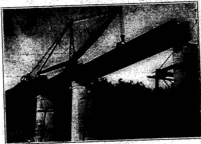
Bridge 104-1, Toronto Terminal Division, Canadian Pacific Ry. Travelling crane placing new span.
