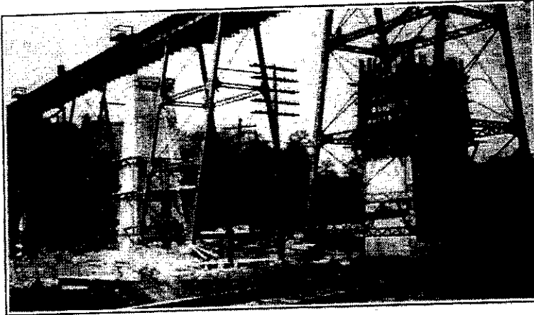
Bridge 105.1, Toronto Terminals Division, Canadian Pacific Ry. Location of new piers with relation to old towers.
