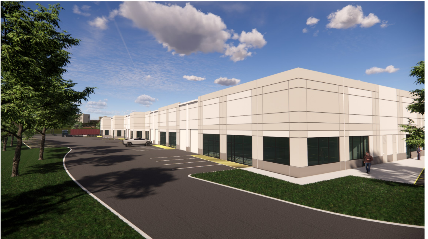
SOUTH LOADING VIEW 1 DTCW LOT 6
