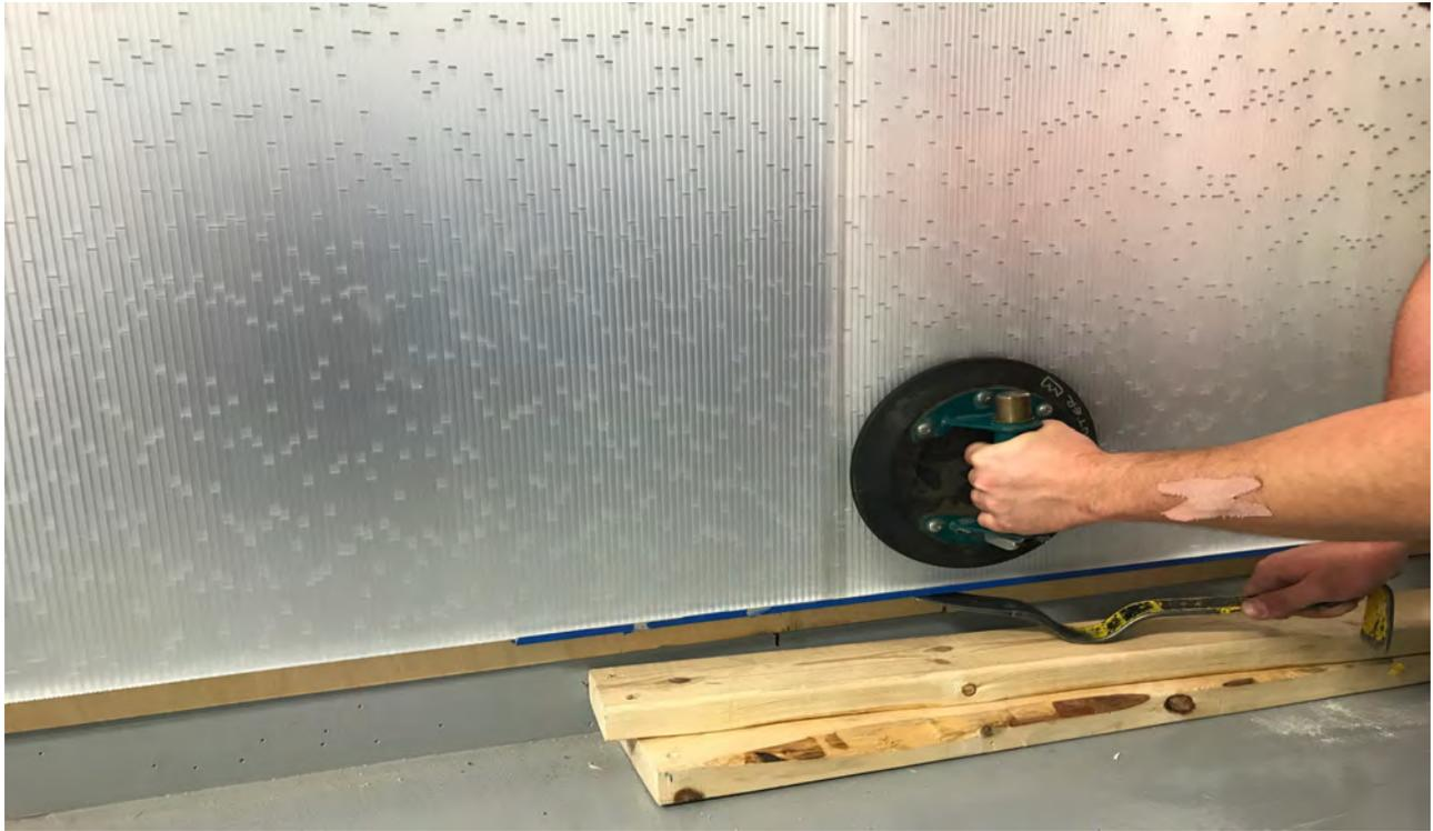
Prybar with gently pressure to ease trim into the panel edges – panel can be pushed/pulled in order to engage trim as needed
