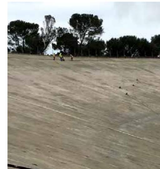
PHOTO C Removing existing batten bar to be stored and reused (4,500 linear feet).
