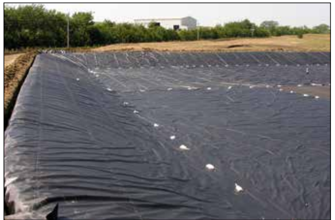
Waste Containment Liner
