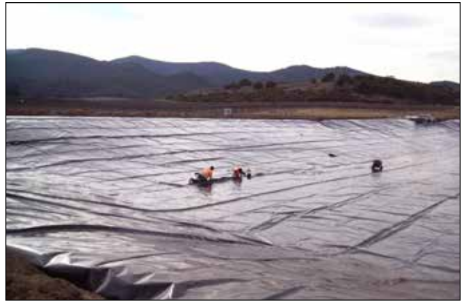
Irrigation Pond Liner
