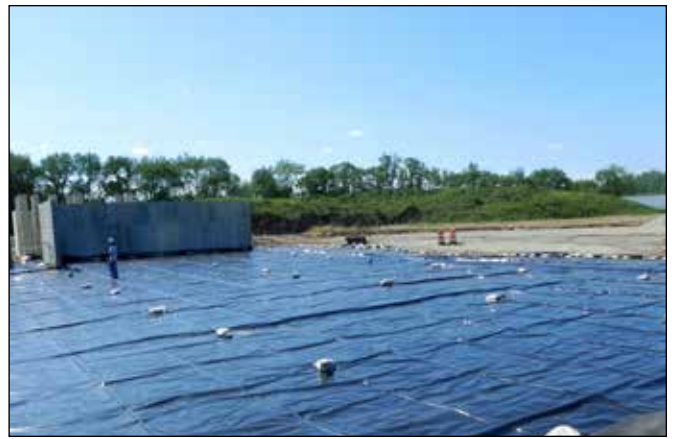
Brownfield Containment Liner
