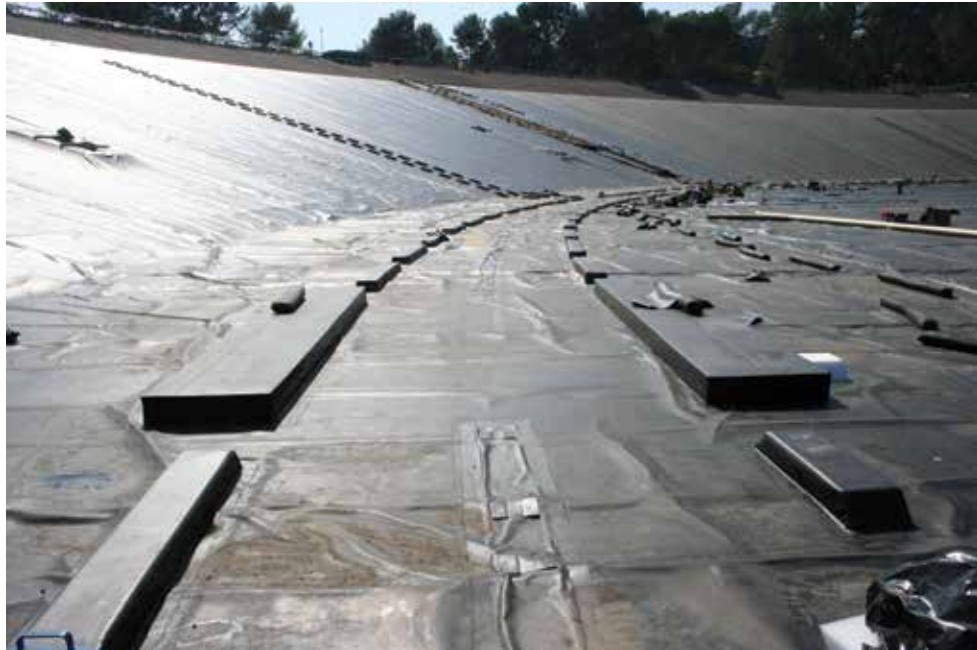
FIGURE 2 Cover installation showing floats and sand tube straps
