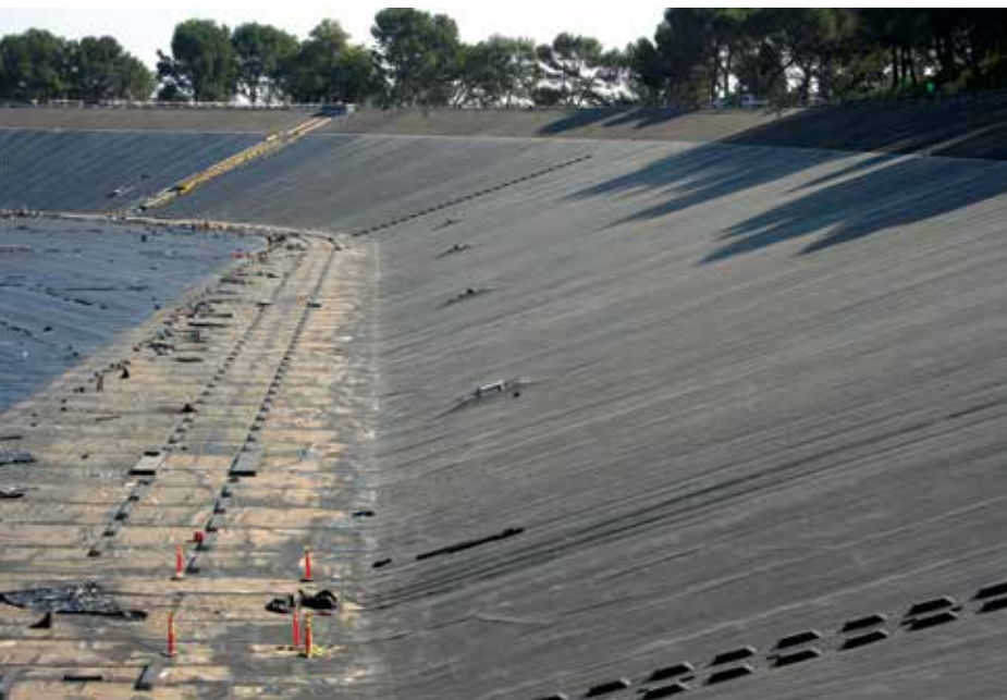
FIGURE 3 South wall with rain collection troughs and hatches
