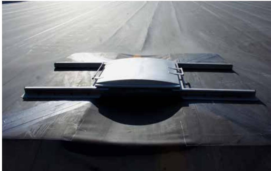
FIGURE 4 Partially installed entry hatch
