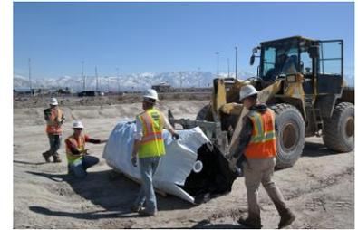
Factory-assembled panel of Absolute Barrier Y30BAC being delivered to jobsite
