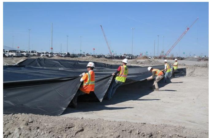
Panel of Y30BAC being opened and installed
