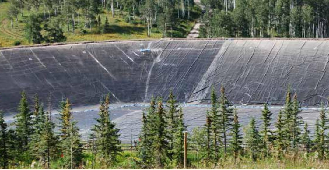
The Raven Modular Construction Model reduces up to 80% of job-site seams for substantial savings in days on site and installation costs by utilizing high quality prefabricated factory panels.
