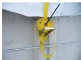
Photo 6 – Webbing tied to wall
