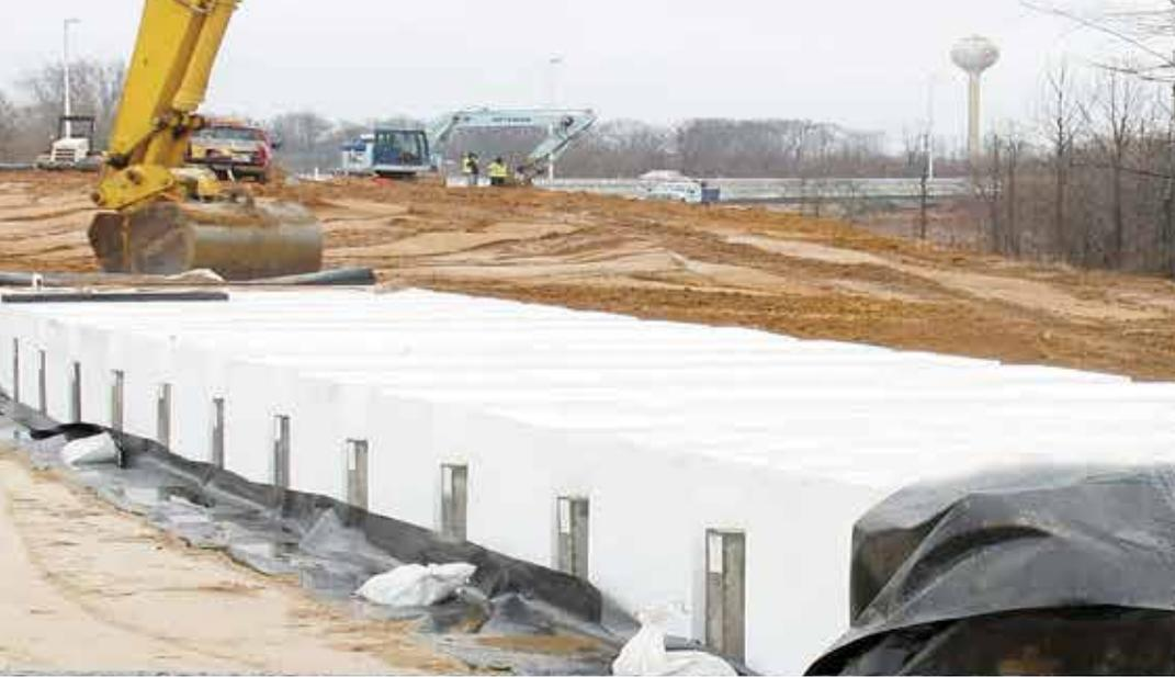
High-tech Absolute Barrier® is a seven layer, co-extruded membrane consisting of a very flexible, linear-low-density polyethylene with a chemically resistant EVOH barrier core layer to provide superior resistance to gas transmission.
