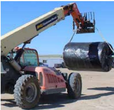
Raven custom panels are accordion folded and rolled tightly on cores for optimized handling and shipping, panels are then easily deployed using proper job-site equipment.
