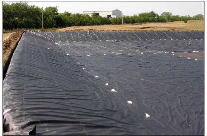
Waste Containment Liner
