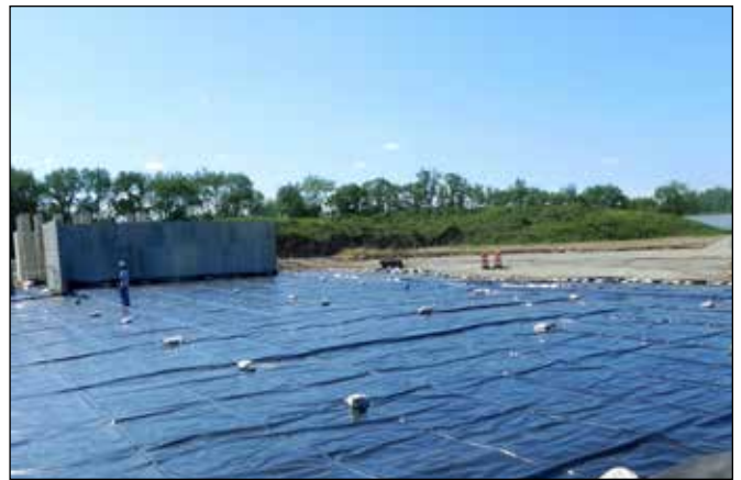
Brownfield Containment Liner
