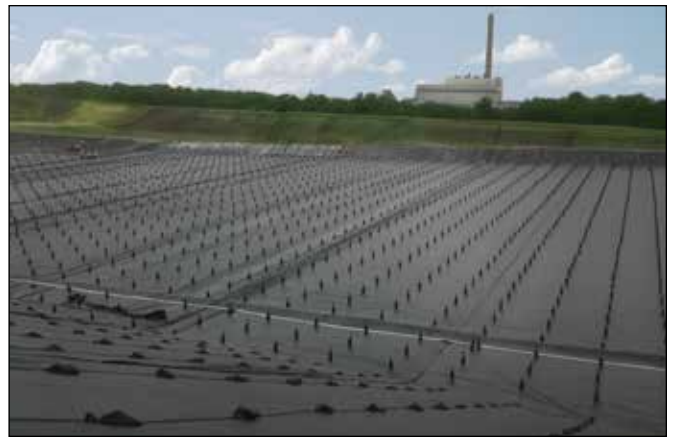
Interim Landfill Cover
