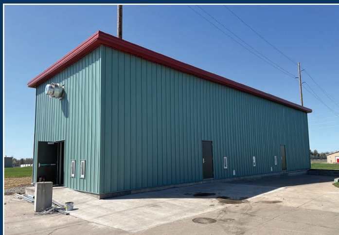
The City of Pella recently built a steel building to enclose two 25,000-gallon fuel-oil storage tanks to ensure reliable generation during cold, winter months.
