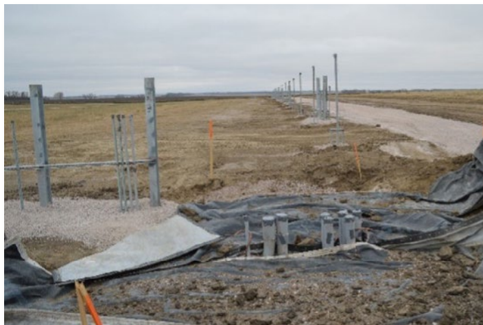
The underground conduit stub-ups are complete.
