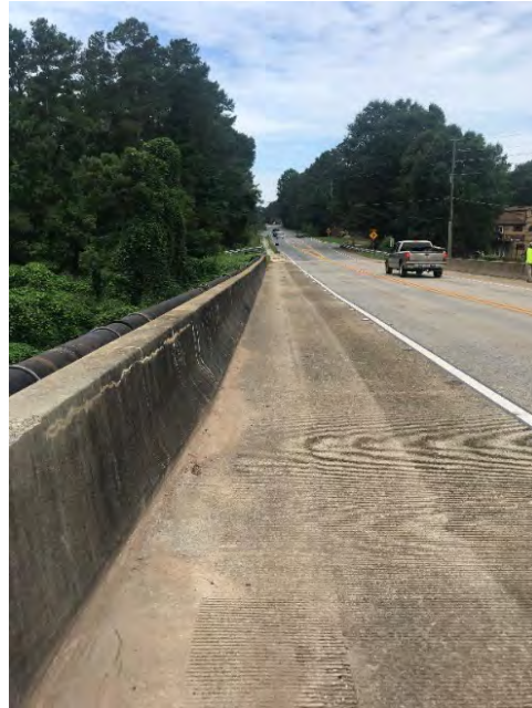
Bridge Contains Both Utilities and Wide Shoulders
