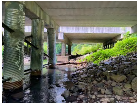
Lower Vertical Clearance And Slope Are Potential Challenges for a Below-Grade Trail Crossing
