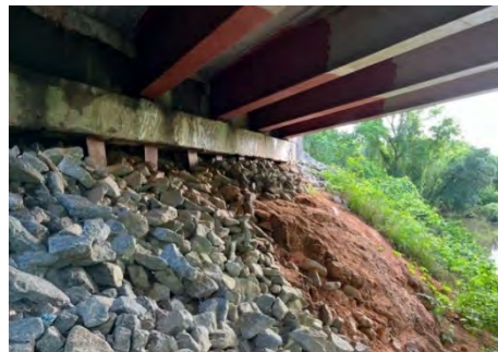
Steep Slopes Underneath the Bells Ferry Road Bridge and Evidence of Erosion
