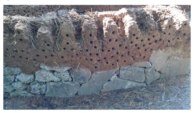
Again, this is an optional step in the process but adds extra integration between layers. The "spine and ribs" technique is more of a North American cobbing technique. It has not been traditionally used in cob construction in Europe or other countries.
