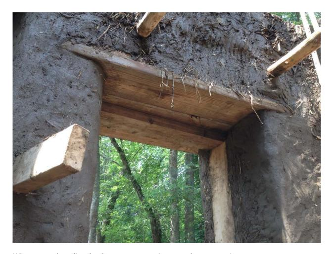
When you place lintels above your openings, make sure to insert temporary supports below them and keep them there until the cob above is completely dried through and solid.
