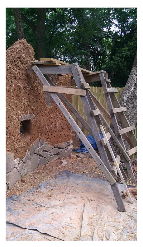
You can also install support beams right through your cob walls as you build them. Then as you reach higher with your walls you can lay boards across these beams and use them as scaffolding. When you're through using them, just cut the beams off flush with the wall and plaster over the exposed wood.
