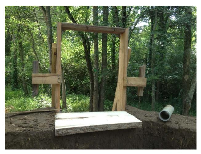
A frame is simply a wooden "box" for your window or door to be attached into. In a conventional stick-framed building, the doors and windows attach into frames just like these. When working with cob walls, the frames are attached into the cob instead of being nailed to the adjacent framing in a stick-frame structure.
