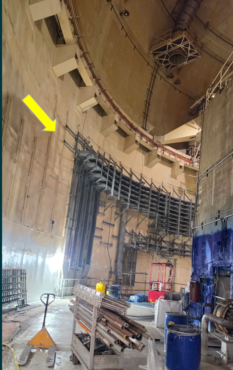
Preparation to remove overhead cable trays in Unit 2 containment on elevation 63'
