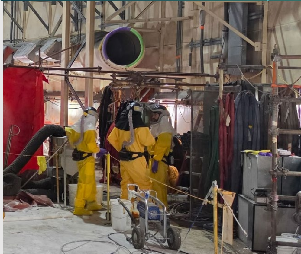
Unit 2 encapsulation (painting for decontamination control) of Reactor Vessel (RV) equipment in preparation of demolition
