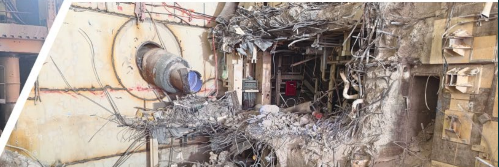
Unit 3 Containment Interior Demolition
