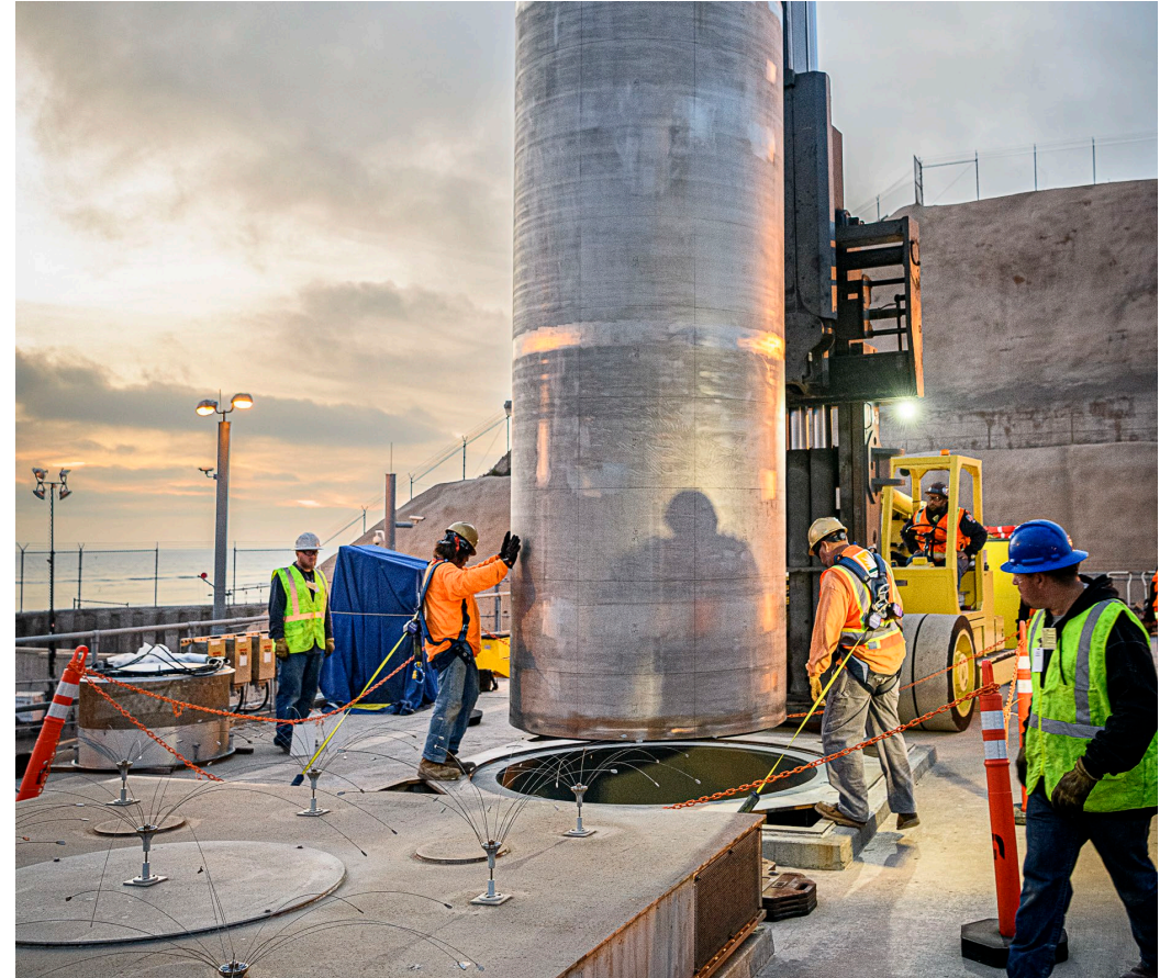
Test canister installation at SONGS
