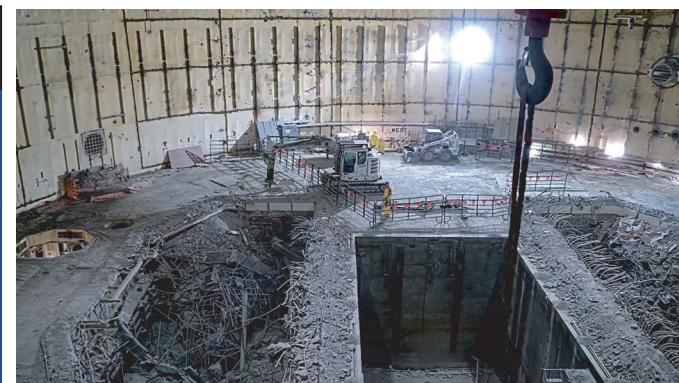
Unit 3 Inside Containment Demolition: The refueling deck and fuel pool area has been emptied and the concrete floor is being rubblized, packaged and shipped offsite for disposal.
