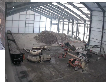
Photo 1 (left): Unit 3 Inside Containment Concrete Demolition
