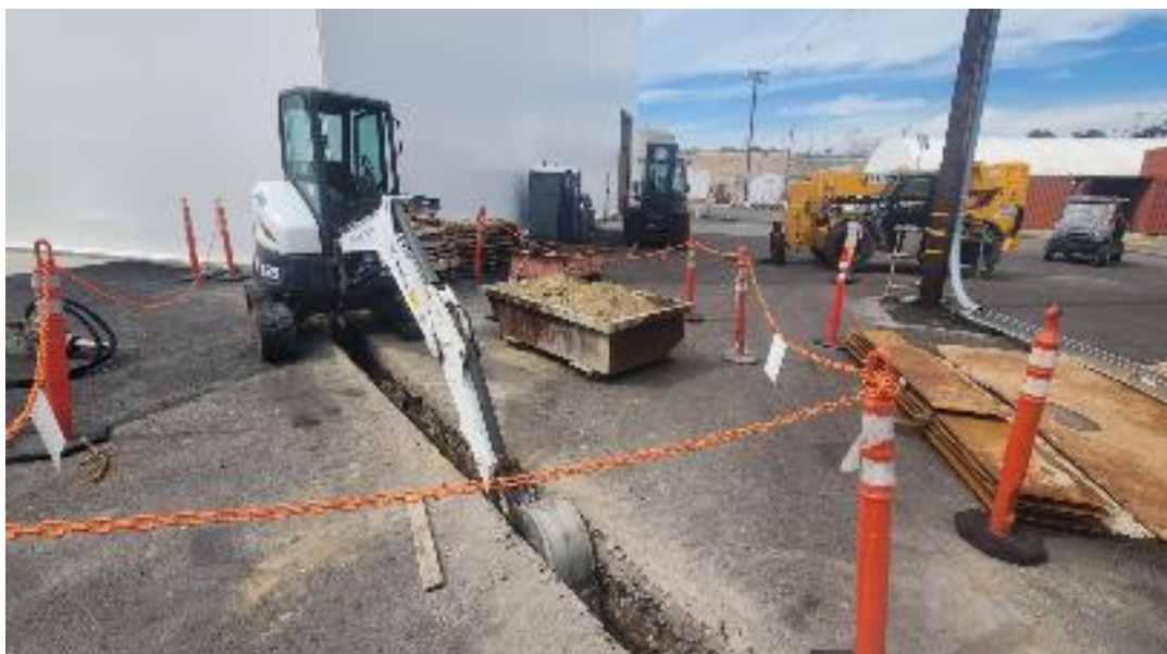
Photo 10 – Trenching for electrical conduit installation for the MHF Building (February 23, 2024).
