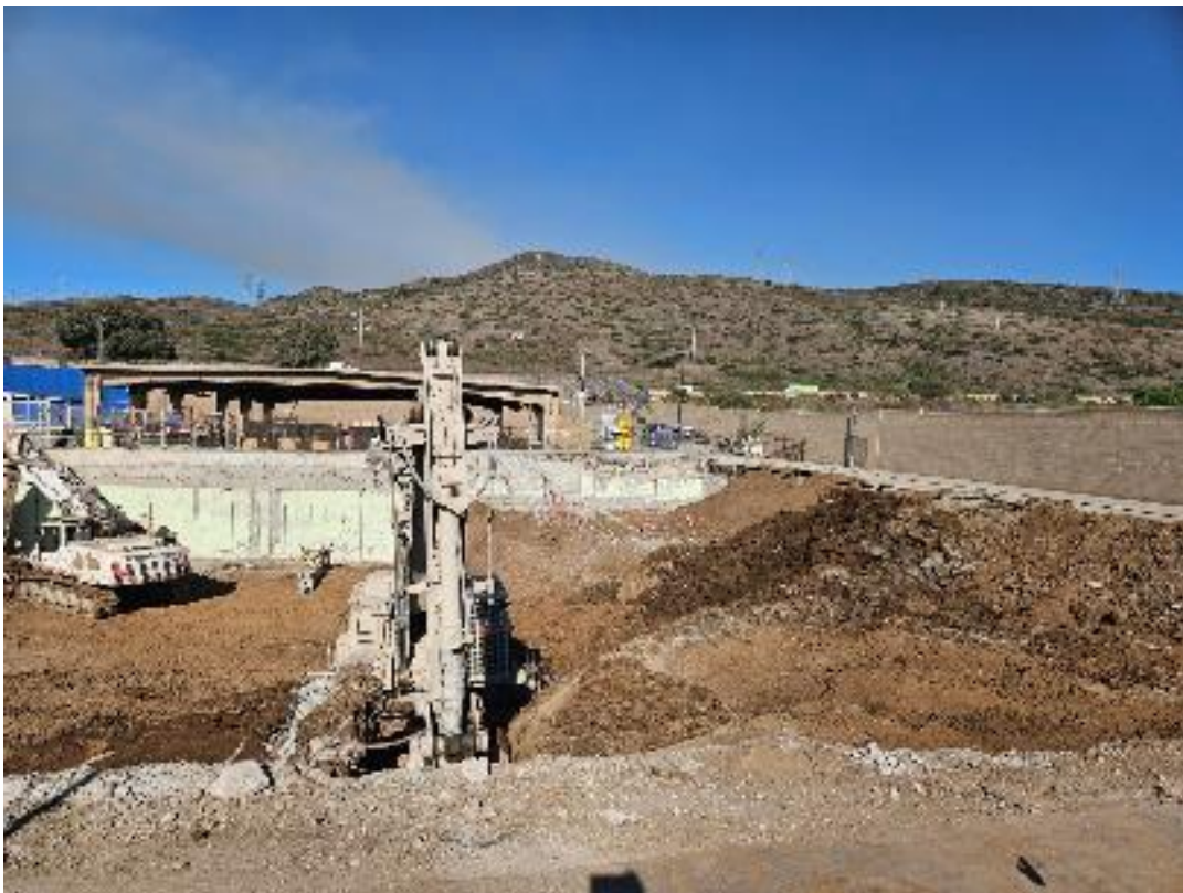
Photo 6 – Completing demolition activities at the MPH Building (November 1, 2023) (photo courtesy of SCE).
