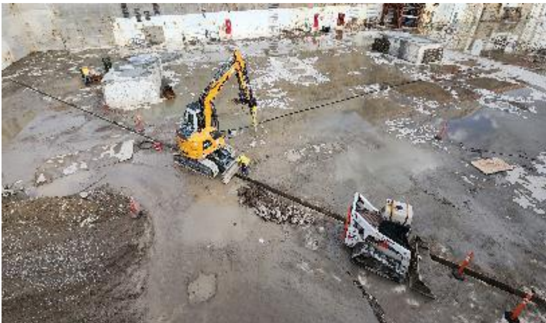
Photo 8 – Trenching for new radiological waste line (November 21, 2023) (photo courtesy of SCE).
