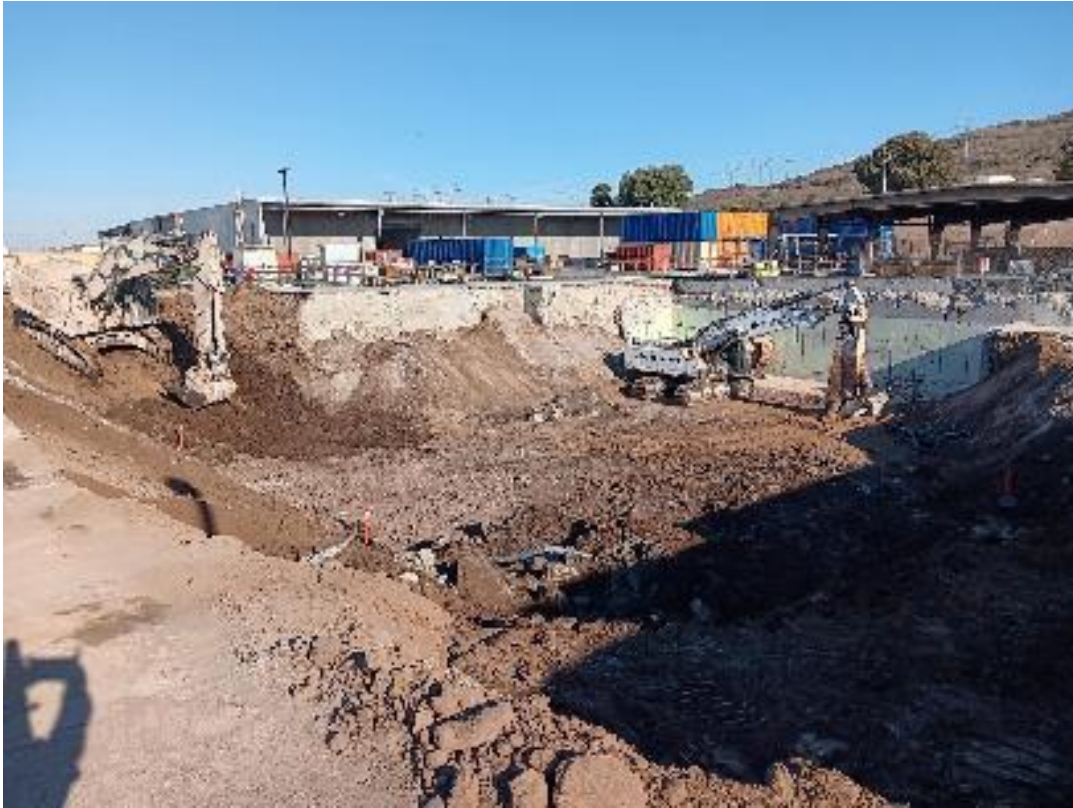
Photo 7 – Completing demolition activities at the MPH Building (November 3, 2023) (photo courtesy of SCE).
