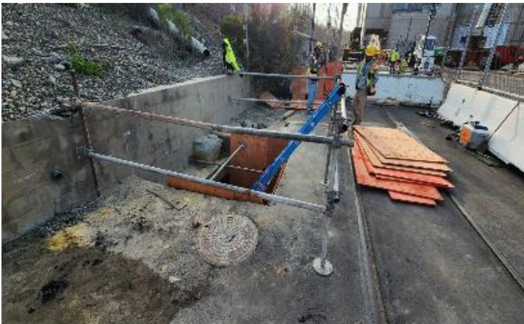
Photo 2 – Isolation of fire hydrant line directly south of the railyard (March 13, 2024) (photo courtesy of SCE).
