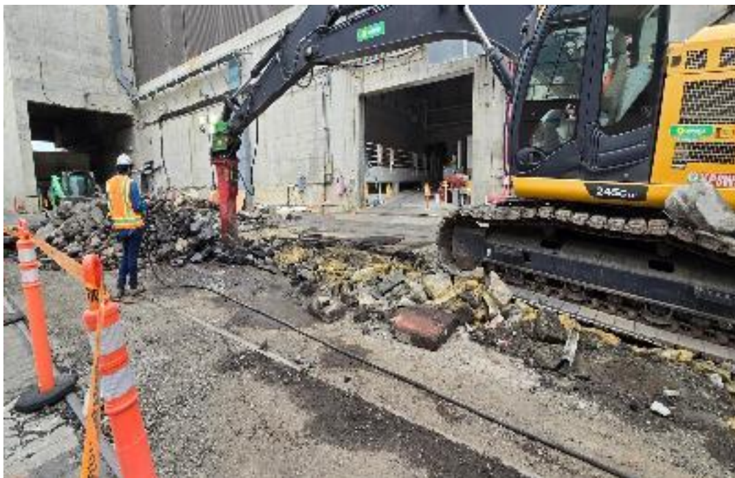
Photo 3 – Installation of new switch rail between Unit 2 and Unit 3 Containment Buildings (June 20, 2024) (photo courtesy of SCE).
