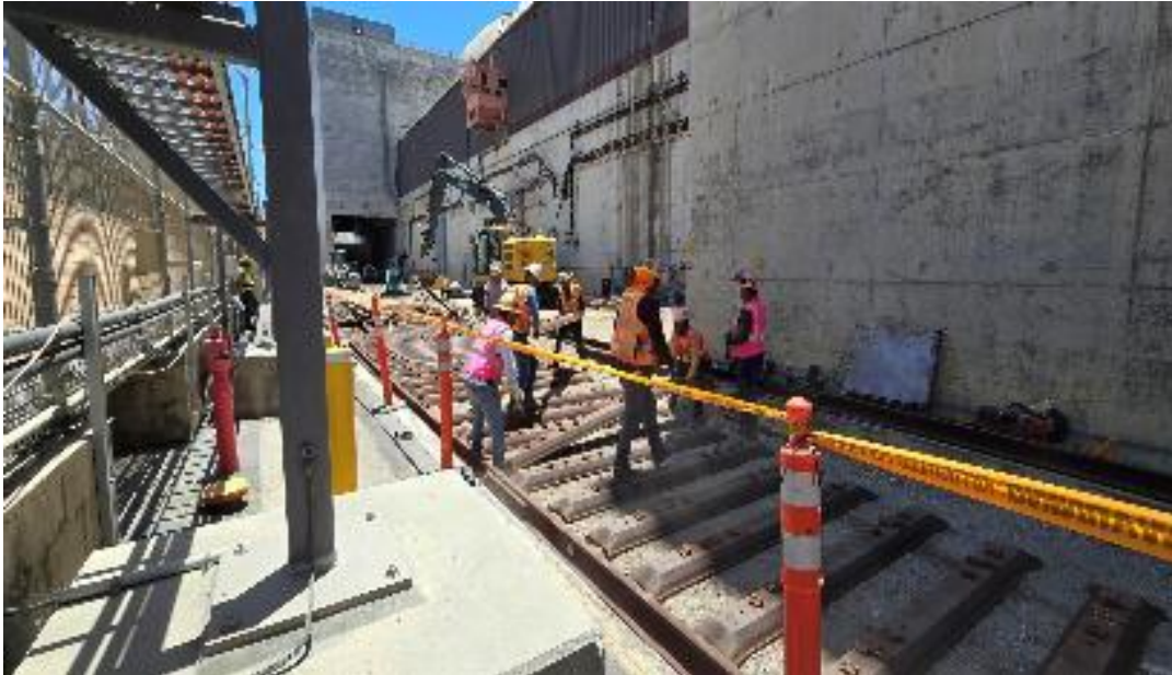
Photo 5 – Installation of new switch rail between Unit 2 and Unit 3 Containment Buildings (June 27, 2024) (photo courtesy of SCE).
