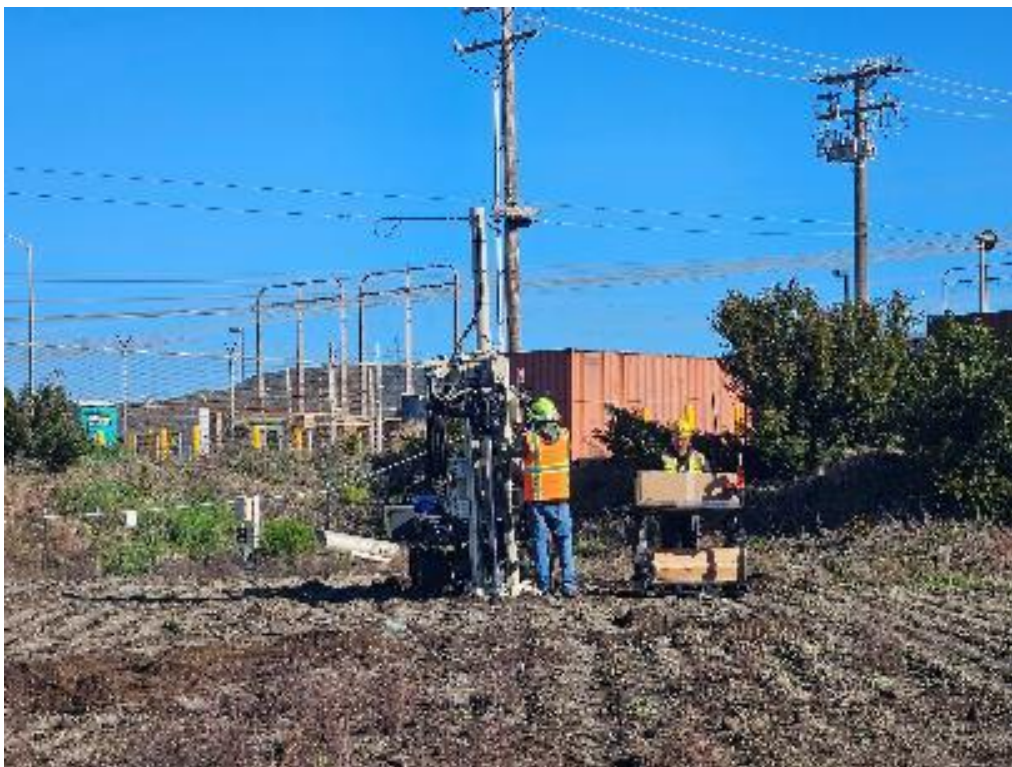
Photo 11 – Soil testing at the MUDA (April 1, 2024) (photo courtesy of SCE).
