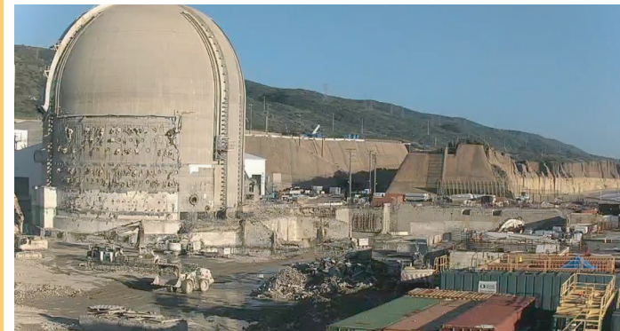
First to go - The area inside and around the Unit 3 containment dome is being cleared in preparation for dismantlement later this year.
