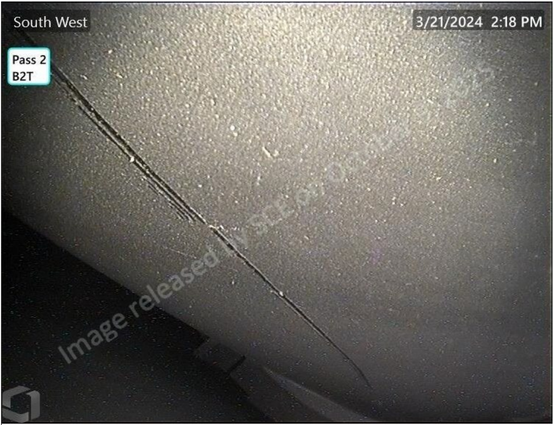
MPC072 Inspection 2024 (close-up)
