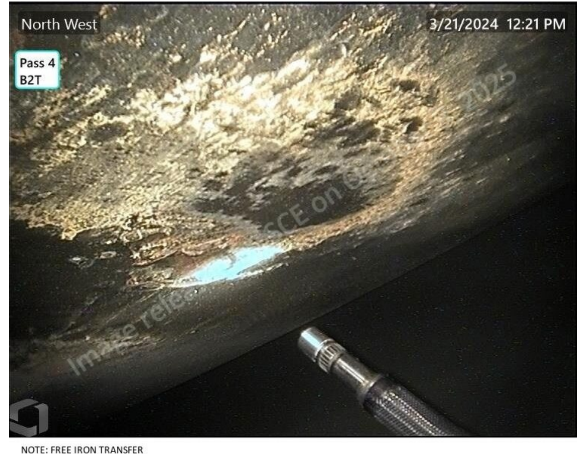
MPC072 Inspection 2024 (close-up)
