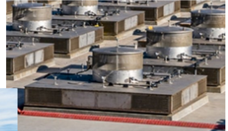
Old outlet vent covers
