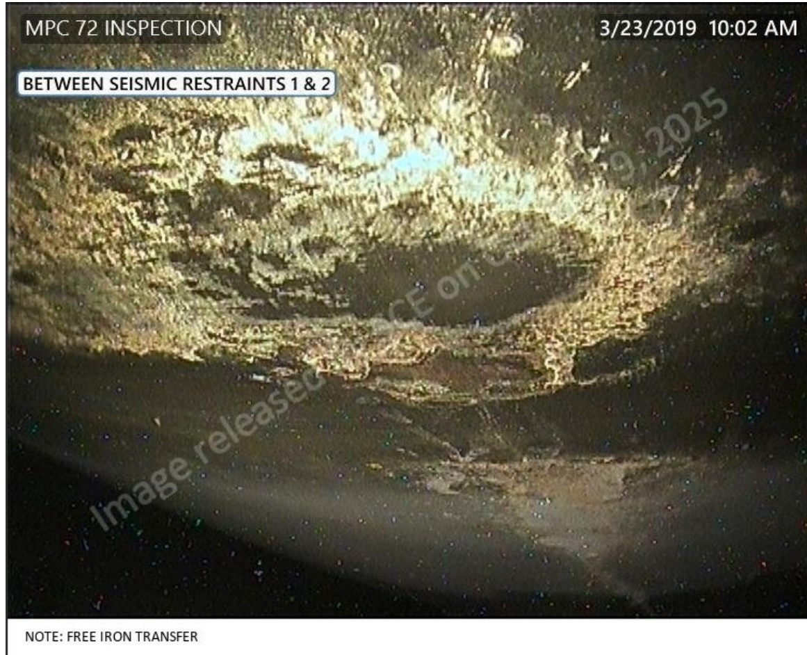
MPC072 Inspection 2019 (close-up)
