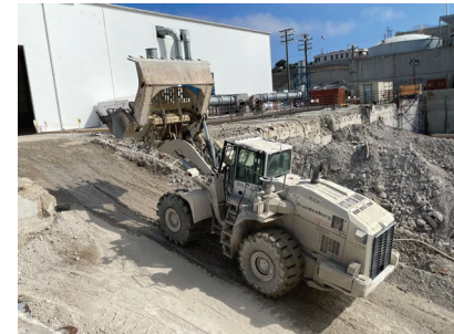
Building debris is moved into the MHF for railcar loading.
