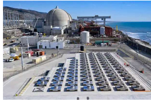
Dry storage for nuclear waste at the San Onofre Nuclear Generating Station (Photo by Jeff Gritchen, Orange County Register/SCNG)
