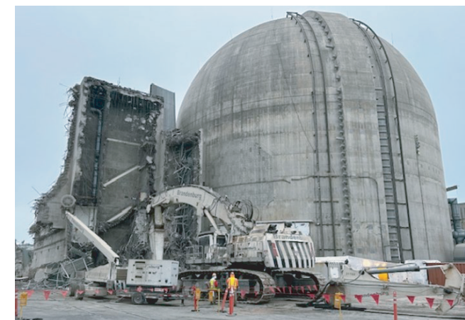
Top Photo: Unit 3 demolition progress
