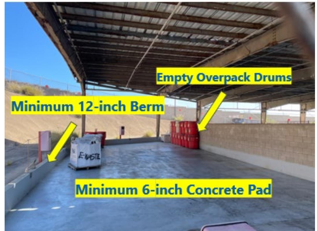
HazMat Area Section A Secondary Containment
