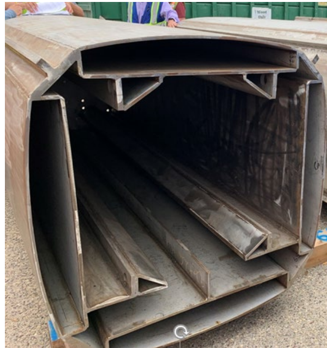
"Furniture," used to arrange and support reactor vessel internals segments, staged for installation in liner.
