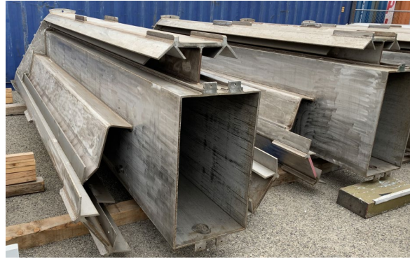
"Furniture," used to arrange and support reactor vessel internals segments, staged for installation in liner.
