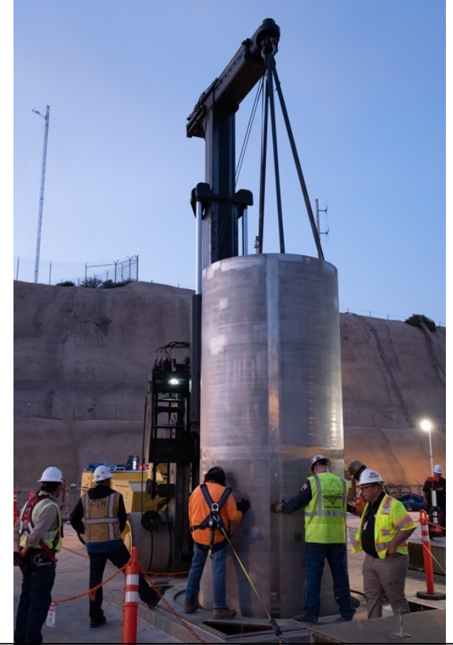
Installation of SONGS Heated Test Canister
