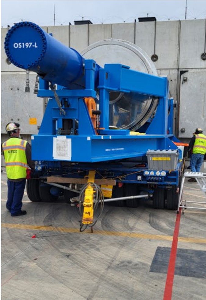
A GTCC canister loaded into a concrete horizontal storage module
