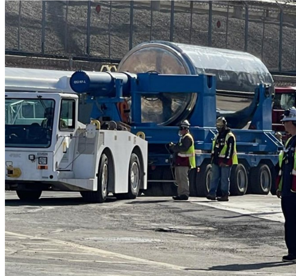
GTCC container being transported from containment to ISFSI
