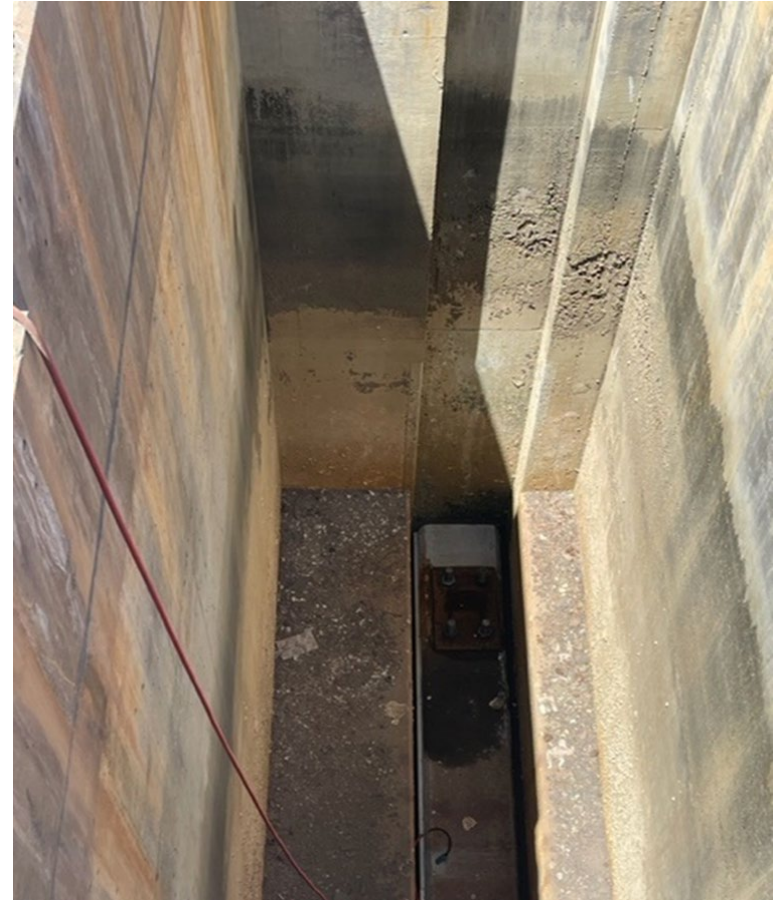
Gate slot (Unit 3 gate 5) with gate installed and sealed. Gates are installed in slots 1, 3 and 5 on Unit 3 side and slots 3 and 5 on Unit 2 side.
