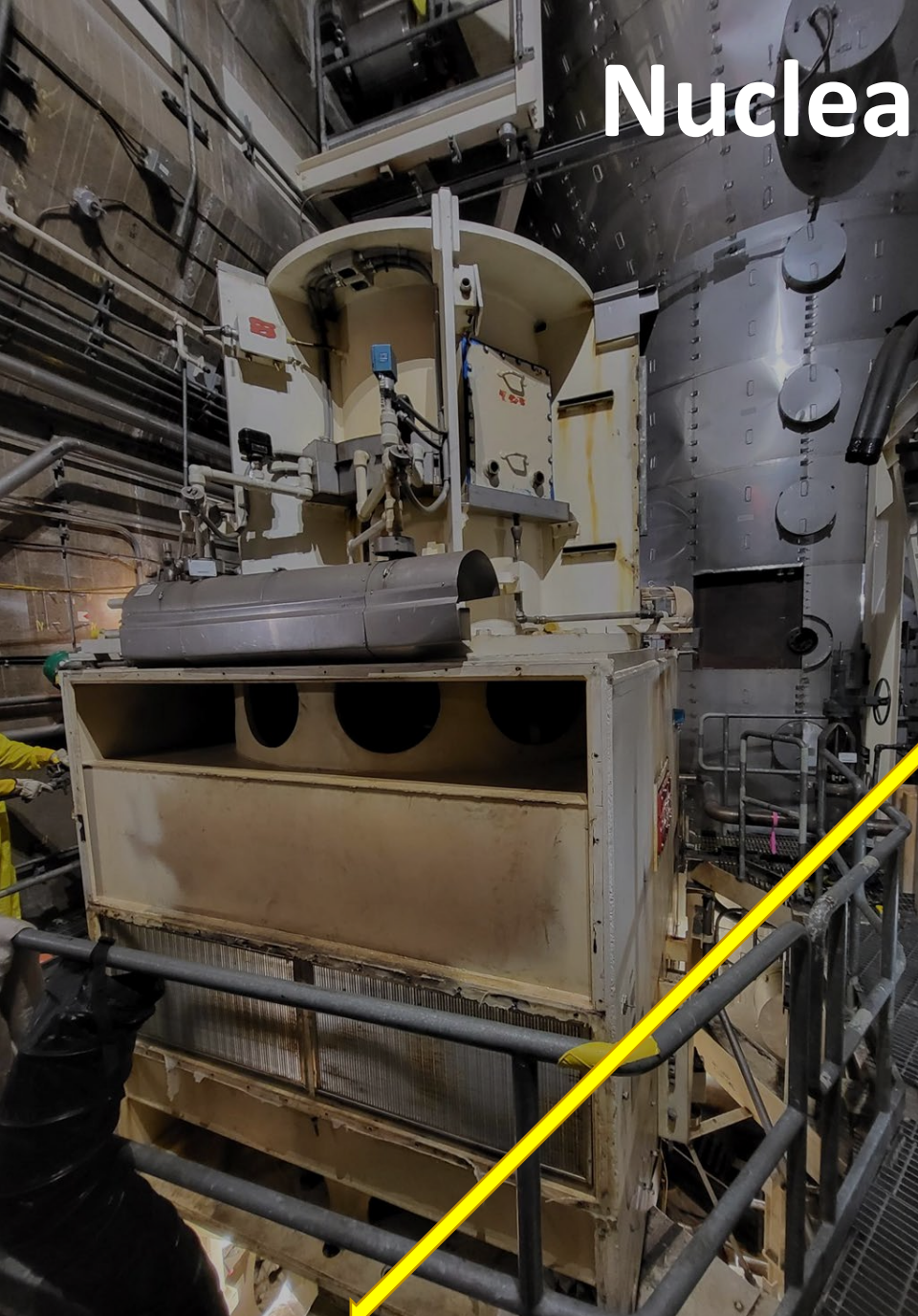
Reactor coolant pump motor interference removal
