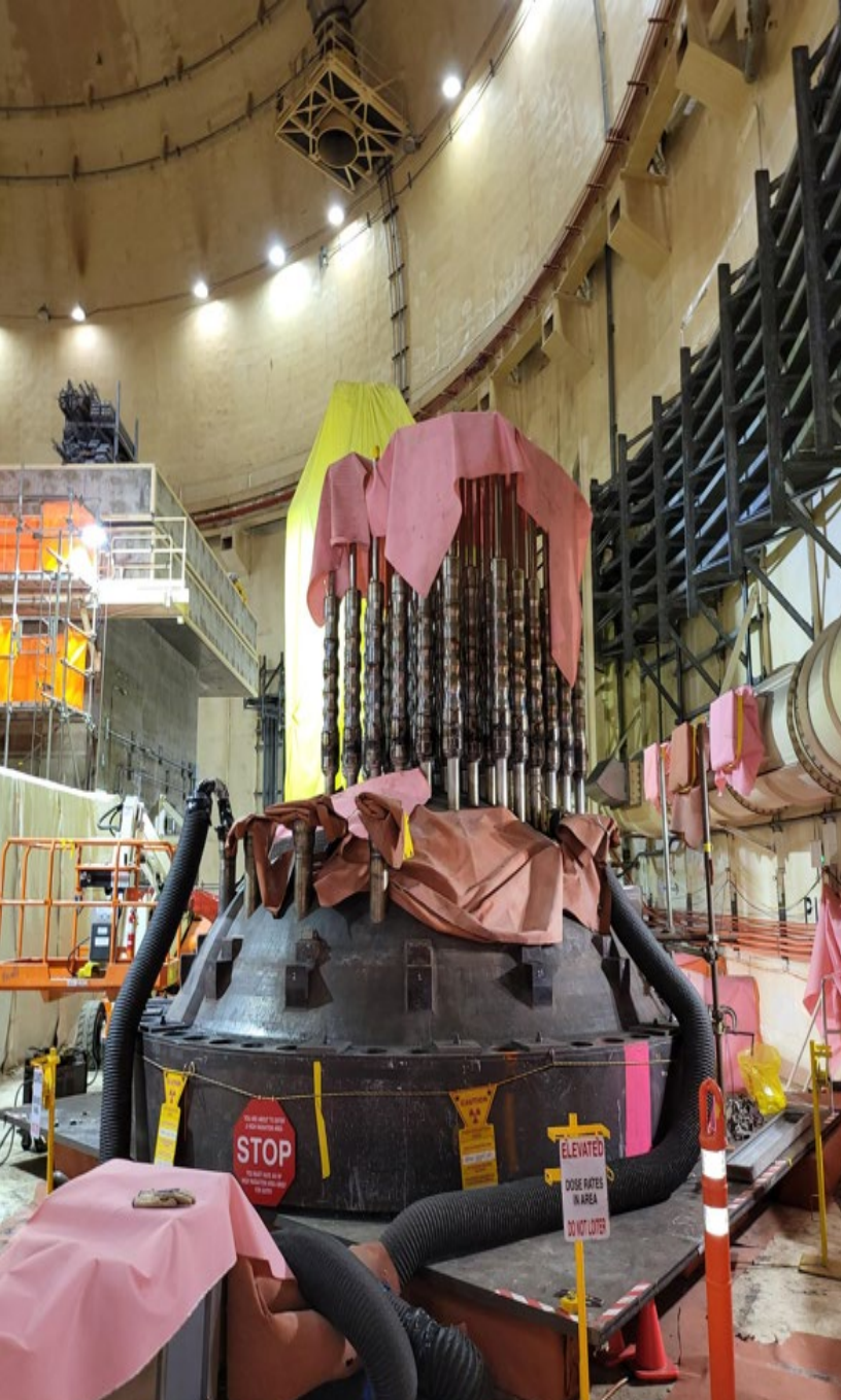
Downsizing Unit 3 reactor head
