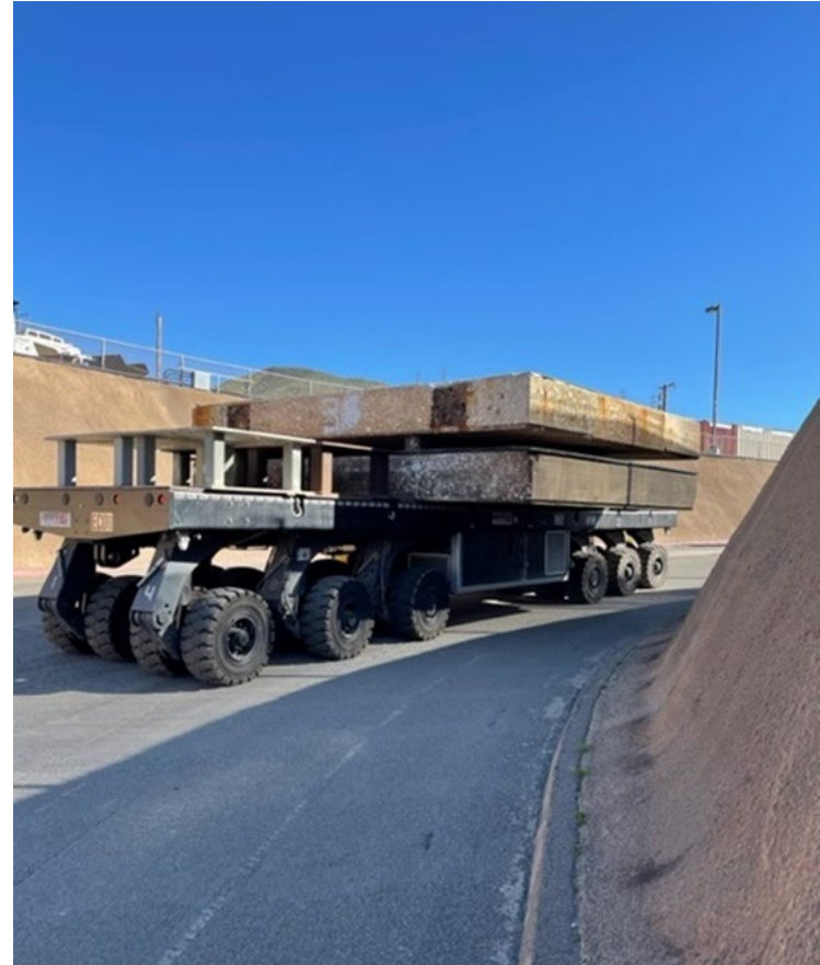
Removed gates being transported to lot 4 on the Cometto self-propelled transporter for future use
