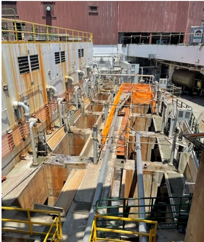
Unit 2 intake forebay with the screens and rakes removed
