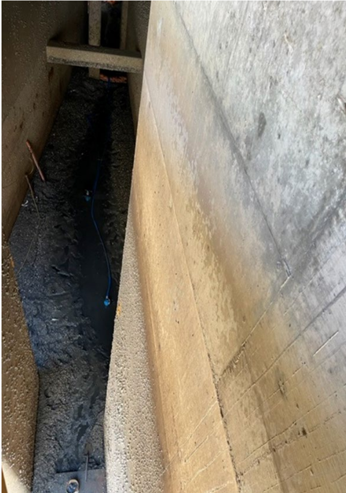
Unit 3 intake forebay dewatered
