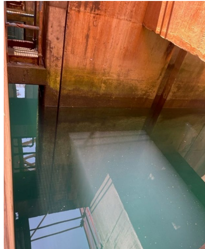
Unit 2 forebay still flooded to ocean level
