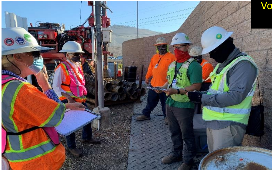
Regulatory visit observing installation of monitoring well
