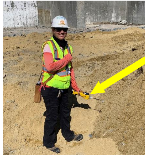
Volatile organic monitoring during soil excavation
