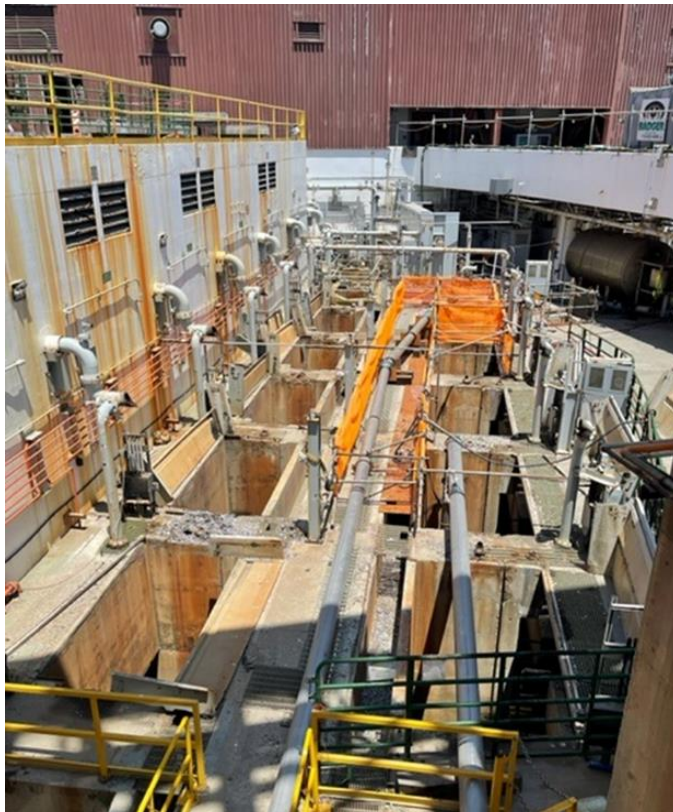
Unit 2 intake forebay with the screens and rakes removed
