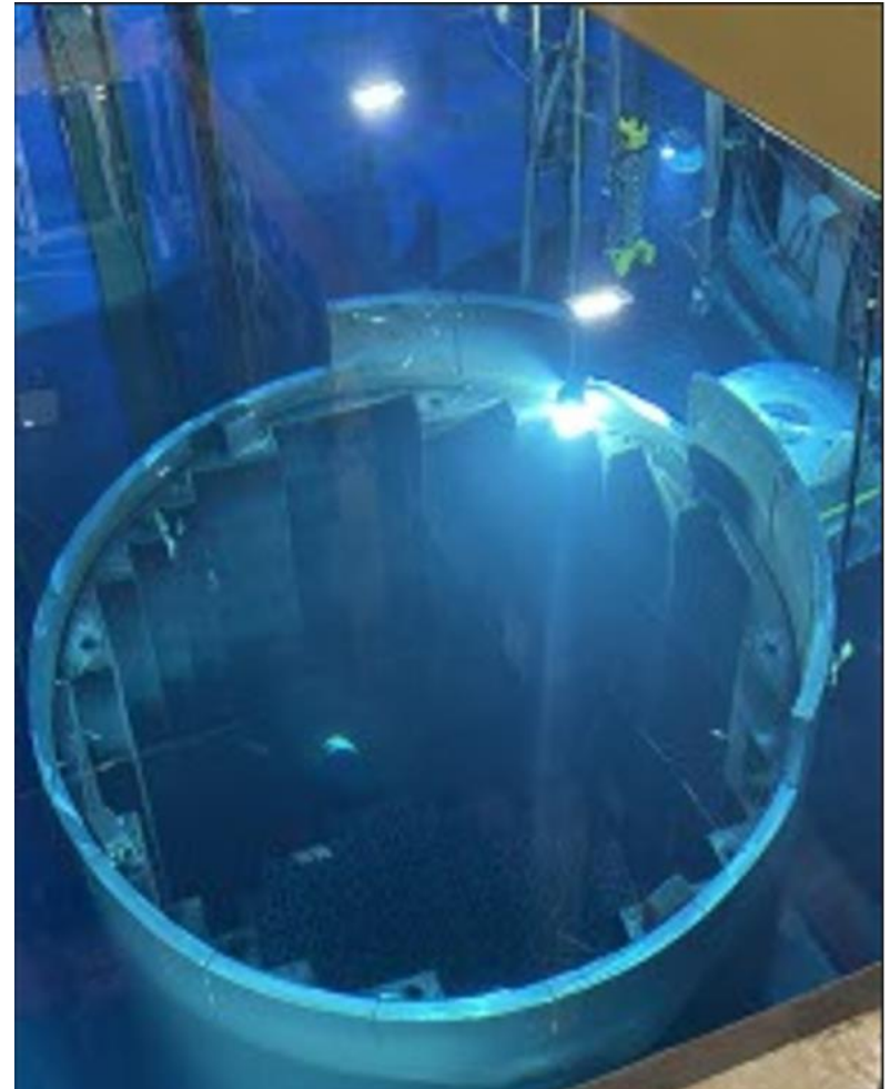
Unit 3 core barrel support C-ring 5 pieces remain
