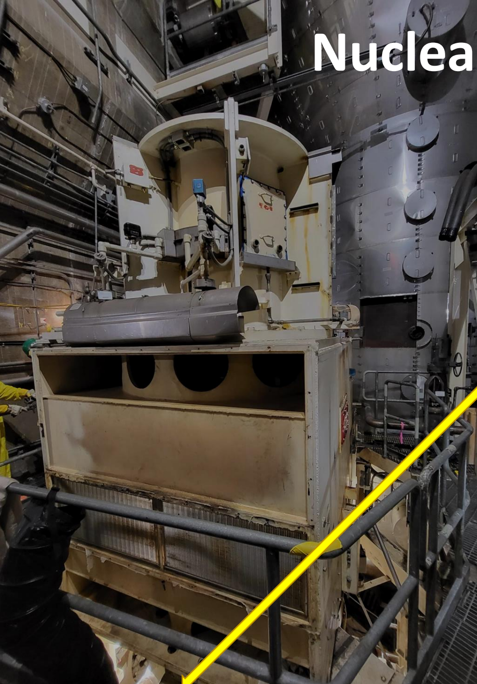
Reactor coolant pump motor interference removal
