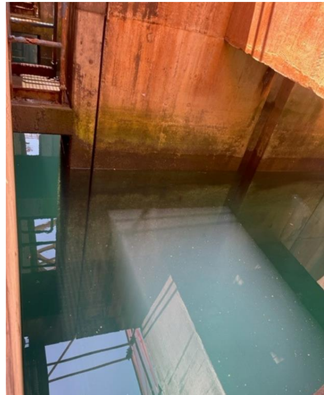
Unit 2 forebay still flooded to ocean level
