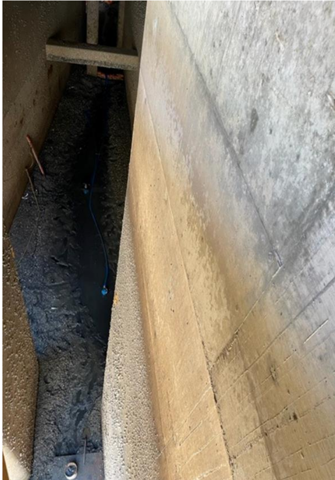
Unit 3 intake forebay dewatered
