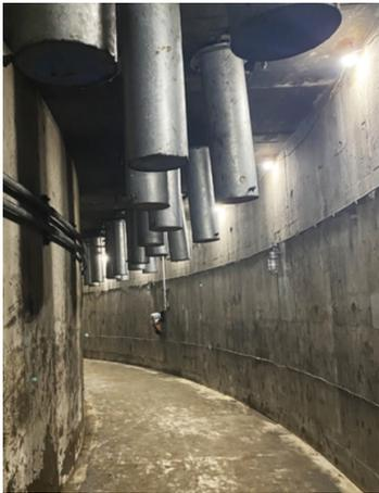
*There are approximately 5,700 miles of tendon strands in each containment dome. The vertical tendons in the containment tendon gallery pictured here are typically 450 feet in length.*
